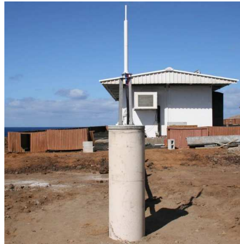
Type II (22%): custom-made tripod on concrete pillar
