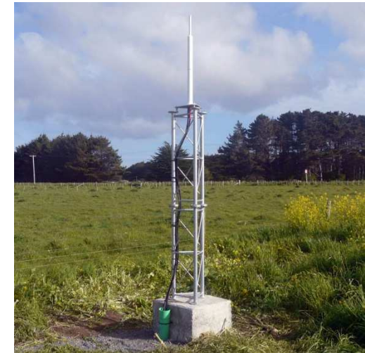
Type III (27%): very rigid steel tower on concrete block
