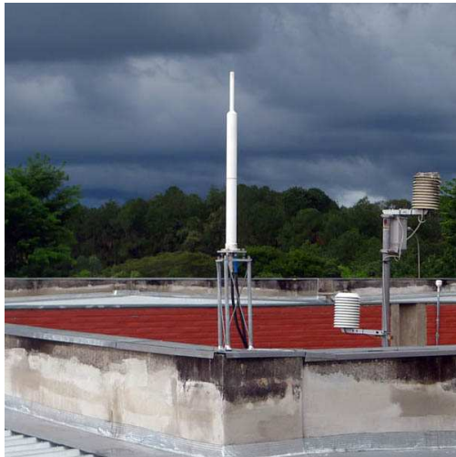
Type I (29%): steel tower on load-bearing wall of a small building
