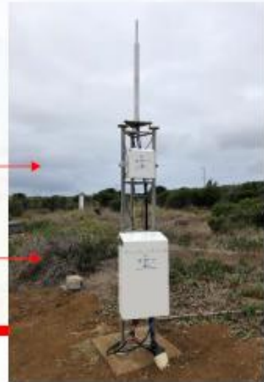
Saint Helena antenna with Leclerc pillar
