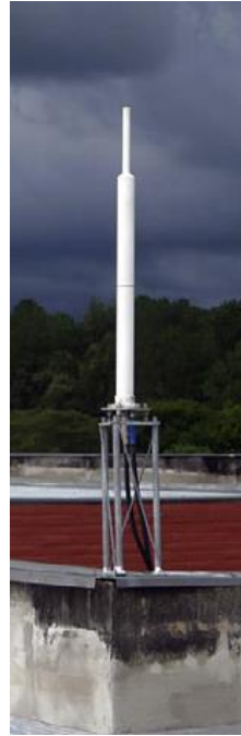
Type I. (CADB, Cacheira). Metal tower on load-bearing building pillar.
