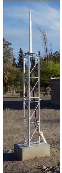
Type III. (SJUC, San Juan) Metal tower on anchored concrete foundation.
