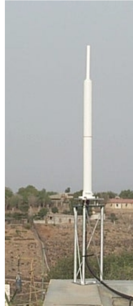
Short tower on building
