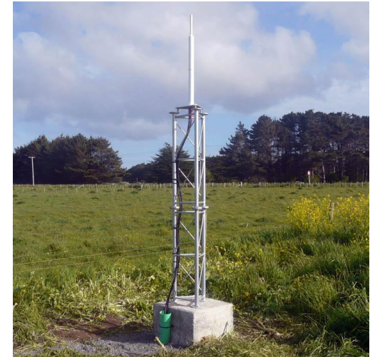
Type III (22%): very rigid steel tower on concrete block
