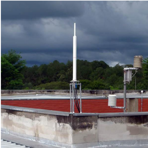
Type I (16%): short antenna support on load-bearing wall of a small building
